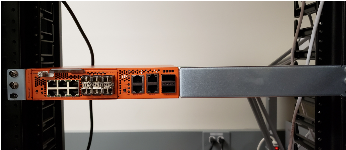
Figure 7 Four-Post Rack Installation (Single Chassis Assembly)
